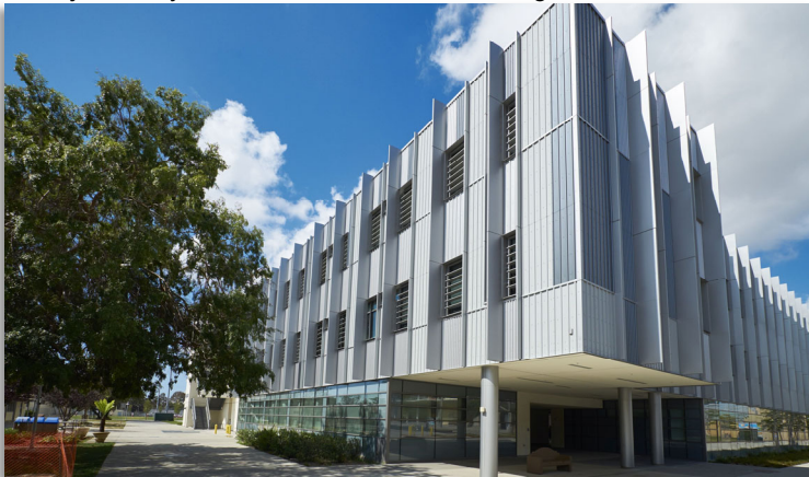
LAHC Science Complex (LEED Platinum)
